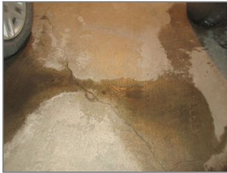
Common settling cracks noted
