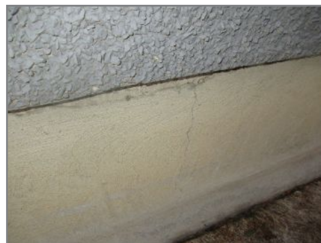
Common settling cracks noted
