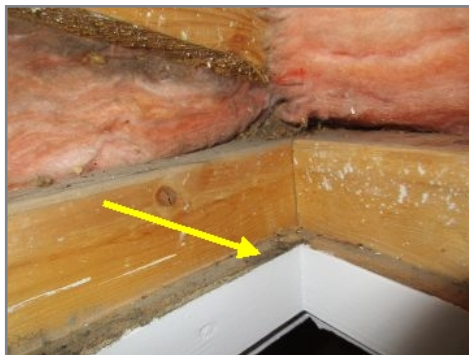
Recommend installing weather stripping around attic hatch
