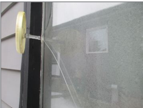
Window pane is cracked
