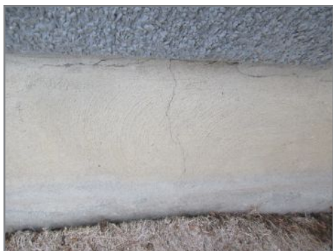
Common settling cracks noted. Recommend monitoring and sealing if required
