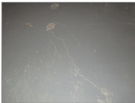
Common settling cracks noted
