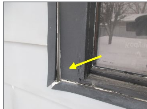
Recommend sealing around this window to keep moisture out of the subwall
