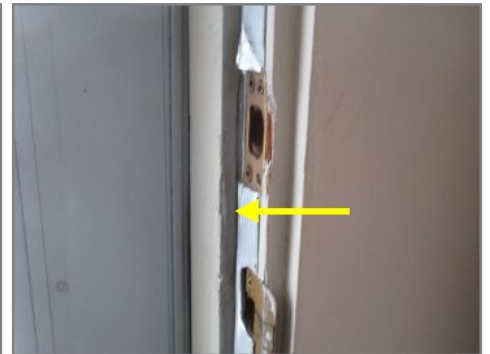
Recommend installing weather stripping on exterior doors
